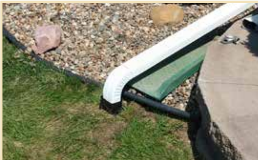
This rain garden is online with downspouts connected to underground drain pipe.
