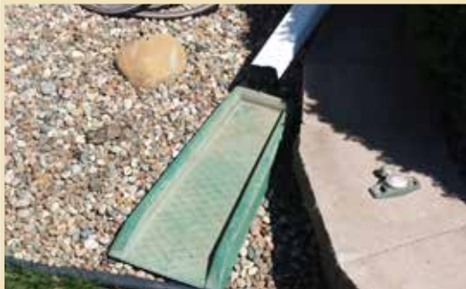
Downspout disconnected to temporarily have rain garden "offline".
