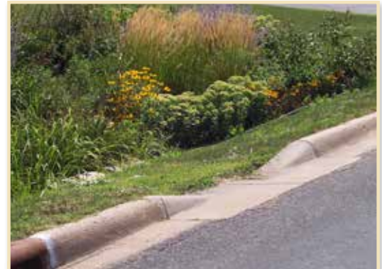
Grass filter strip used for pre-treatment area.
