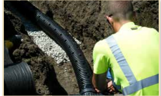
Placement of perforated subdrain.
