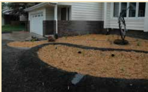
Rain garden berms under construction.
