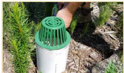
Overflow structure extending to the top of the ponding depth.
