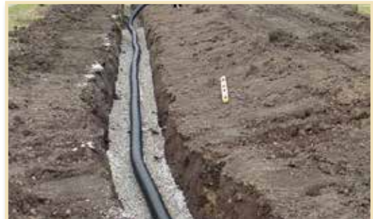
HDPE subdrain pipe in an enhanced rain garden.
