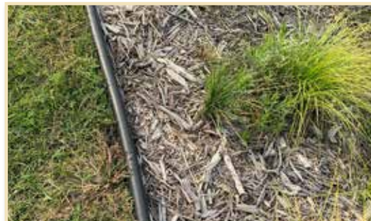
Plastic landscape edging along the perimeter of a rain garden.
