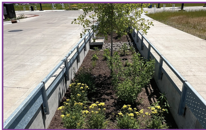
Bioretention cells with trees require a different soil mixture.
