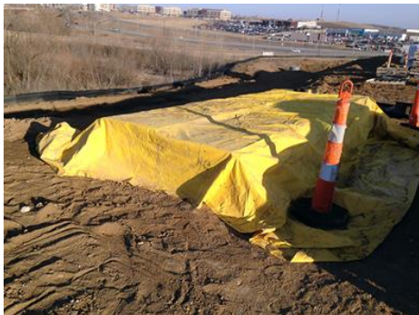
Cover materials using tarps or plastic sheeting to prevent precipitation from contacting construction site materials. Direct work crews to replace material stockpile covers at the end of the day and before rain. Photo credit: Barry Toning, Tetra Tech
