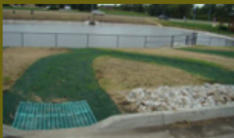
*Rolled Erosion Control Blankets offer excellent cover, especially in areas with concentrated flows and on slopes.*
